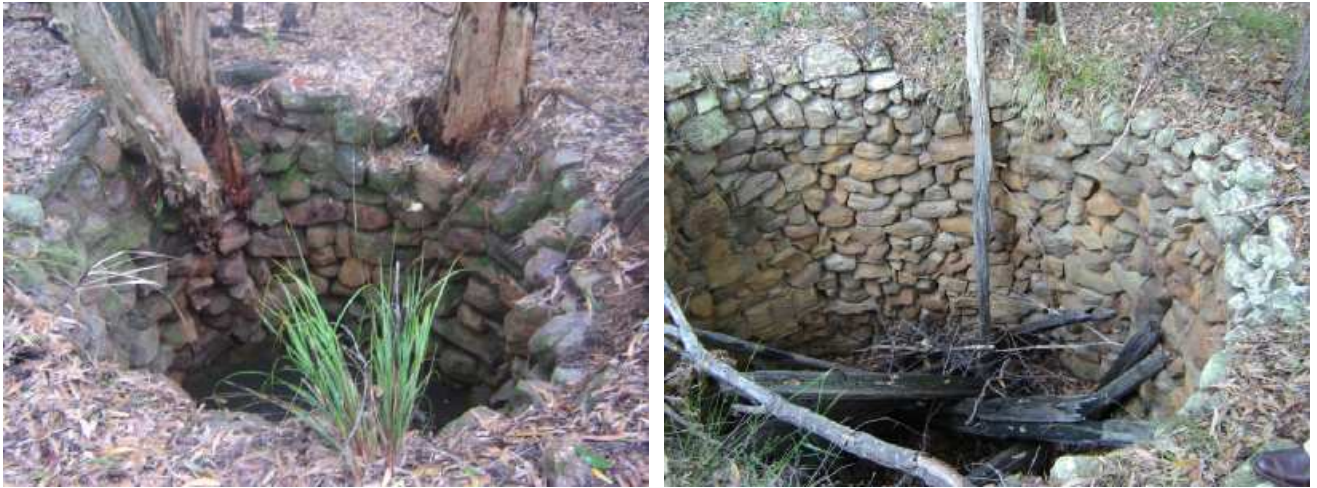
Figure I-16.2 Examples of stone lined wells
