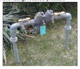
**Medium risk** - Any condition, device or practice within the water supply system and its operation which could endanger health. In this instance, double check valves are used. *Example of double check valve (testable)*
