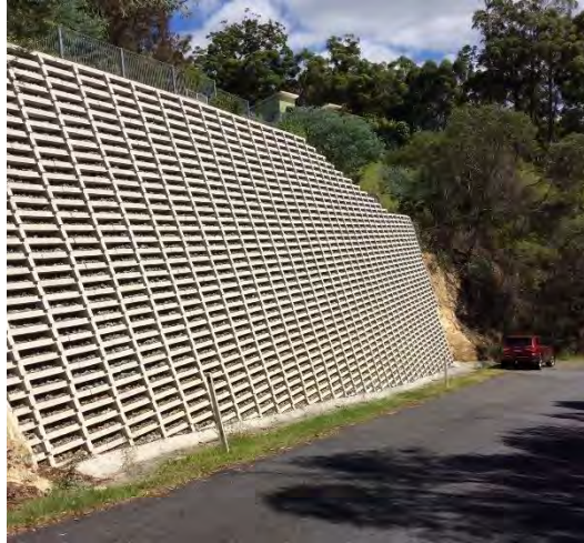
Figure 2- Retaining Wall without Vegetation
