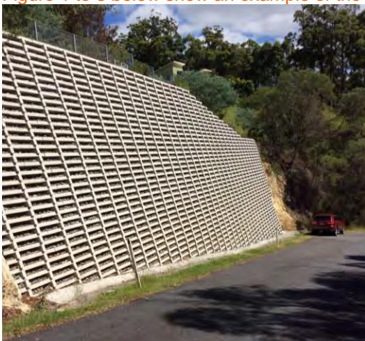
Figure 1- Retaining Wall without Vegetation
