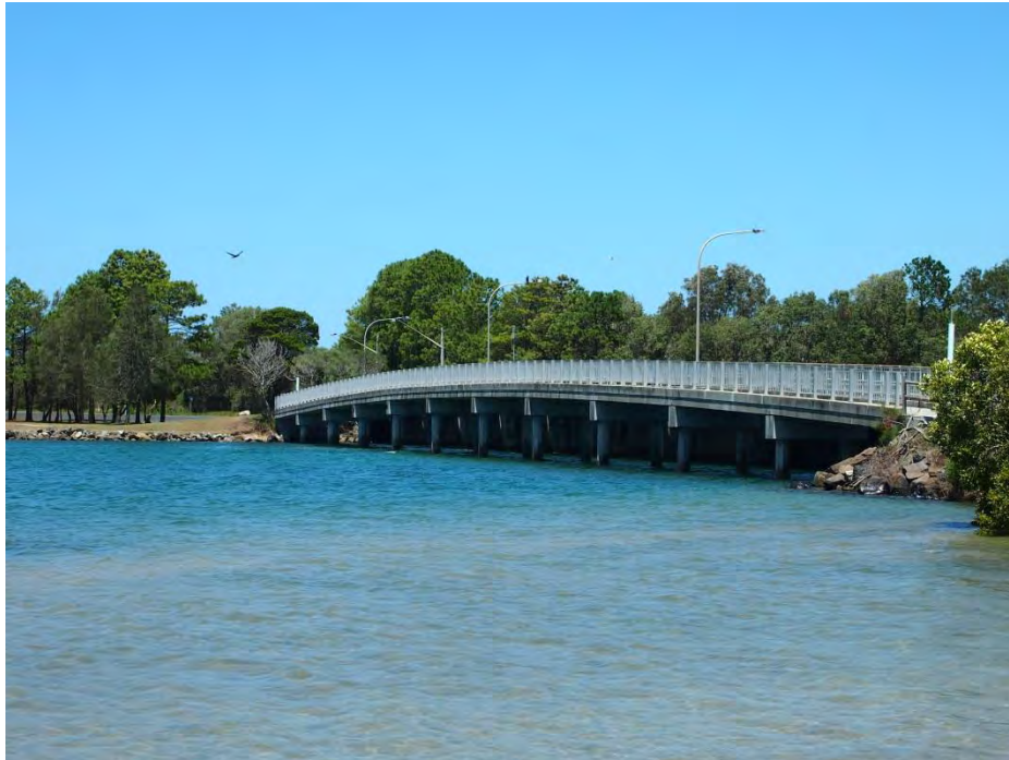
Figure 2-4 Elm Street Bridge at Evans Head
