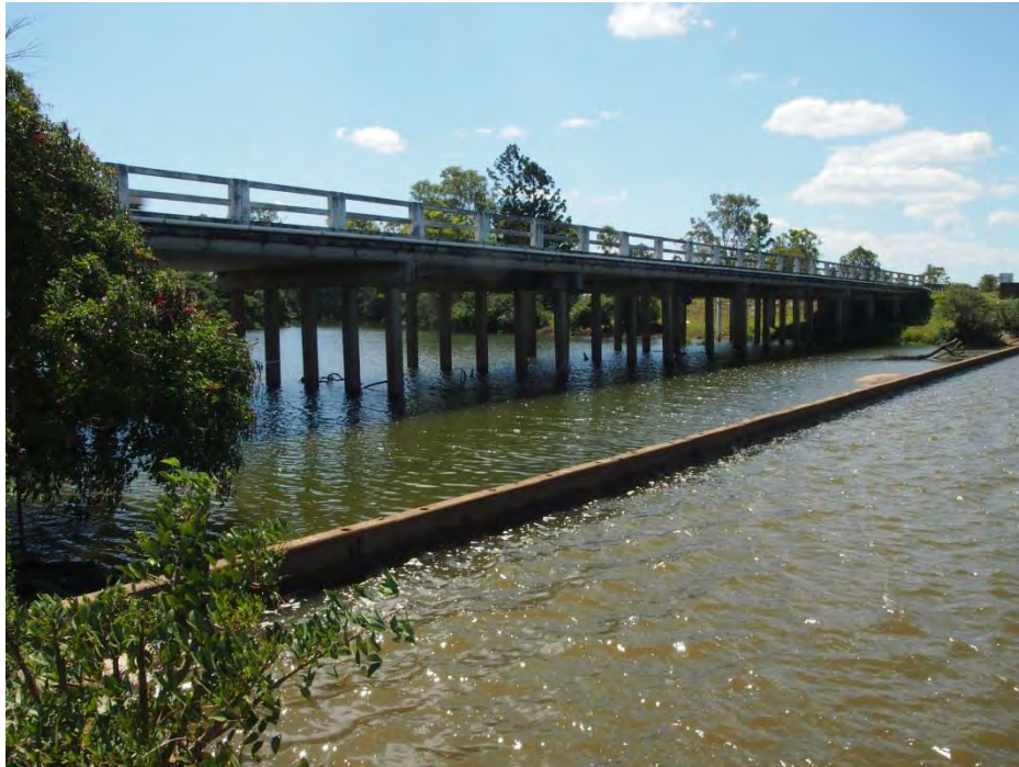
Figure 2-2 Tuckombil Canal Weir and Pacific Highway Bridge (Tuckombil Canal in the foreground, Rocky Mouth Creek in the background)
