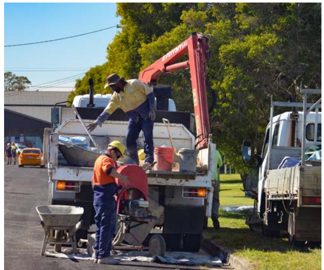
Maintaining infrastructure and assets
