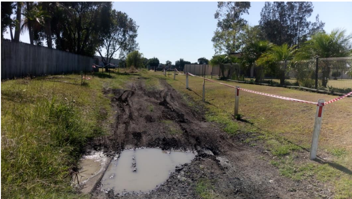
Kent Street Casino – Lack of road and stormwater drainage
