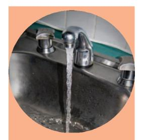
Discoloured water occurs occasionally in all water supply systems. It is most commonly caused when there is a sudden increase or change in direction of water flow through pipes.
