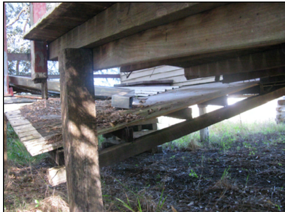
Figure 2.10: Collapsed and damaged non-original verandah on the canteen (Converge Heritage + Community).
