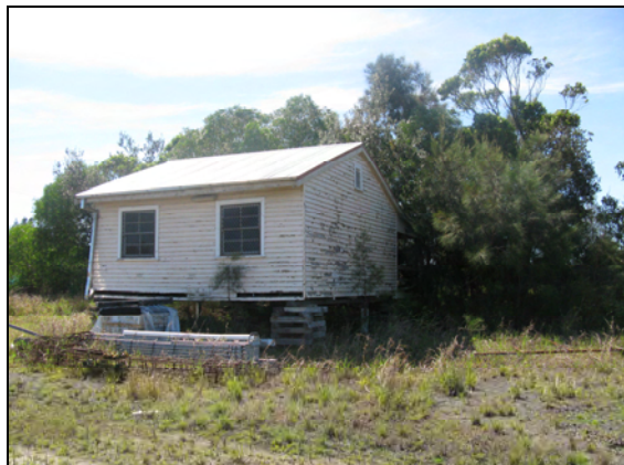
Figure 2.12: Canteen building showing damaged paint and temporary props (Converge Heritage + Community).
