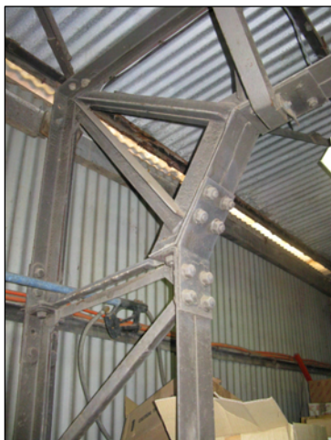
Figure 2.19: Portal frame detail at ceiling (Converge Heritage + Community).
