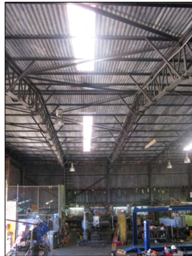
Figure 2.18: Works depot hangar internal portal frames (Converge Heritage + Community).
