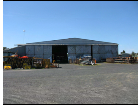
Figure 2.16: Works depot hangar with intact doors showing characteristic external cross-bracing (Converge Heritage + Community).
