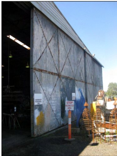
Figure 2.17: Works depot hangar doors and door tracks (Converge Heritage + Community).
