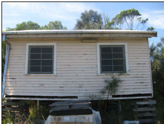
Figure 2.11: Canteen building with damaged weatherboards (Converge Heritage + Community).
