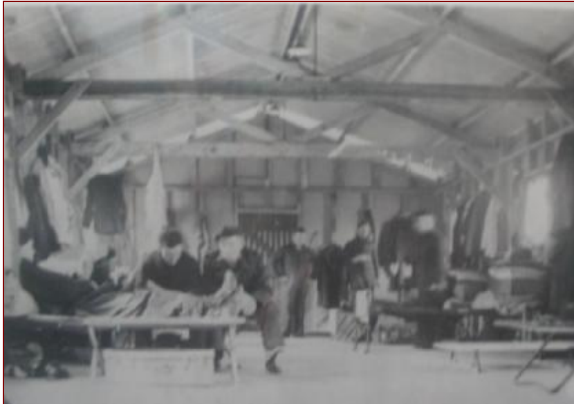
Figure 4.20: Photo of trainees in their accommodation hut at Evans Head Aerodrome. Note the exposed roof trusses, exposed wall and ceiling linings and temporary camp beds.
