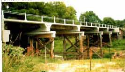
BYRON CREEK BRIDGE - FOR BYRON SHIRE COUNCIL
