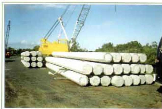
COMPLETED PRESTRESSED OCTAGONAL PILES WAITING DELIVERY
