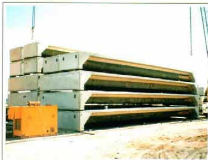
COMPLETED DOOLAN DECK MODULES WAITING DELIVERY.
