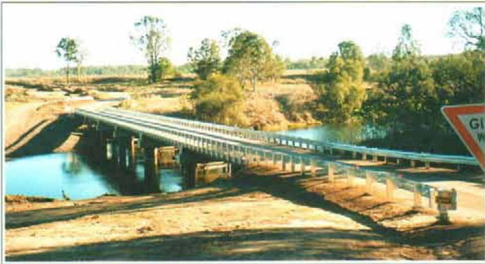
◀ BURTONS BRIDGE ESK SHIRE COUNCIL
